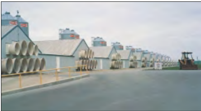
Figure 1. Typical environmentally controlled layer house. (00-CN-0601)
